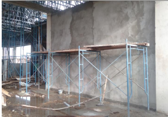
Gambar 6 Perancah Besi Scaffolding
