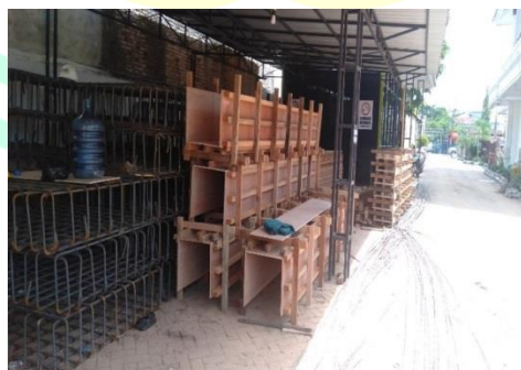
Gambar 1 Bekisting Balok 30/50
